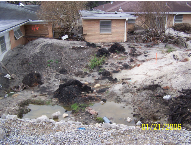
Figure 32. Sand deposits and peat blocks (black) behind homes on Pratt Drive at the North breach of the London Ave. Canal.
