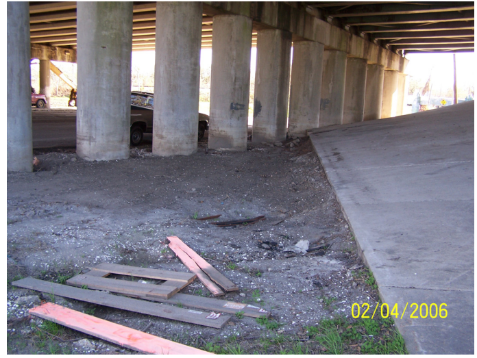
Figure 46. Erosion around the support structures for I-610 near Orleans Canal on Marconi Ave (Stop 6).
