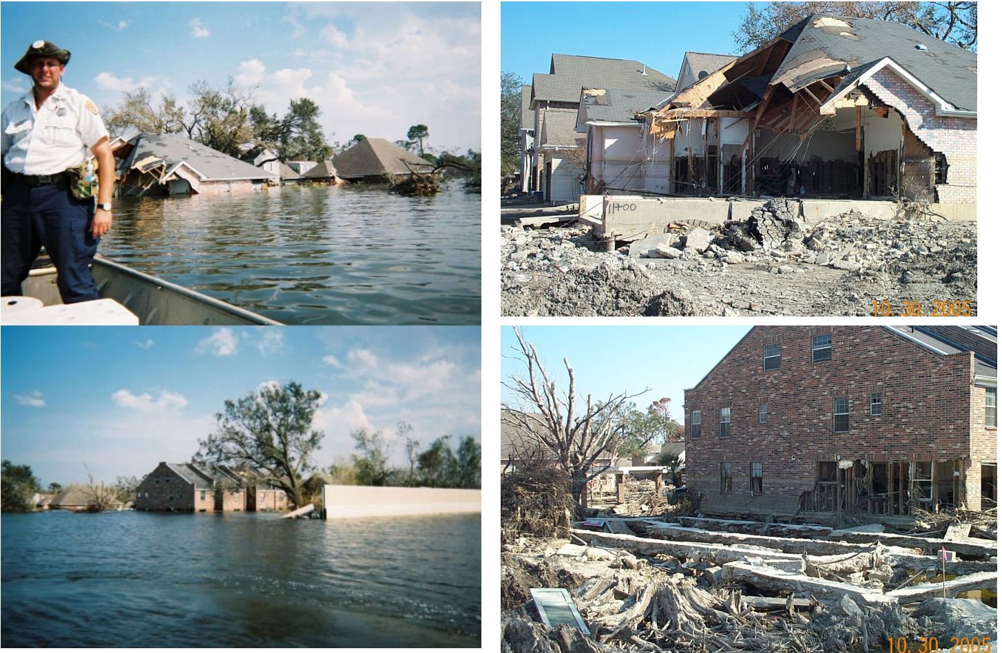
Figure 43. Comparison of water levels on Sept. 1, 2005 (photos on left by Kevin Himmel), with water lines on same structures indicate lines left by standing water are about 1.5 to 2 feet lower than the maximum water level. Note large block of peat in photo at the upper right. In photo at lower right, note the chainwall foundation of a house that was removed by the burst of water when the levee was breached and the cypress stump from a tree that was probably cut down 100 years ago when this Lakeview neighborhood was reclaimed from the cypress swamp.
