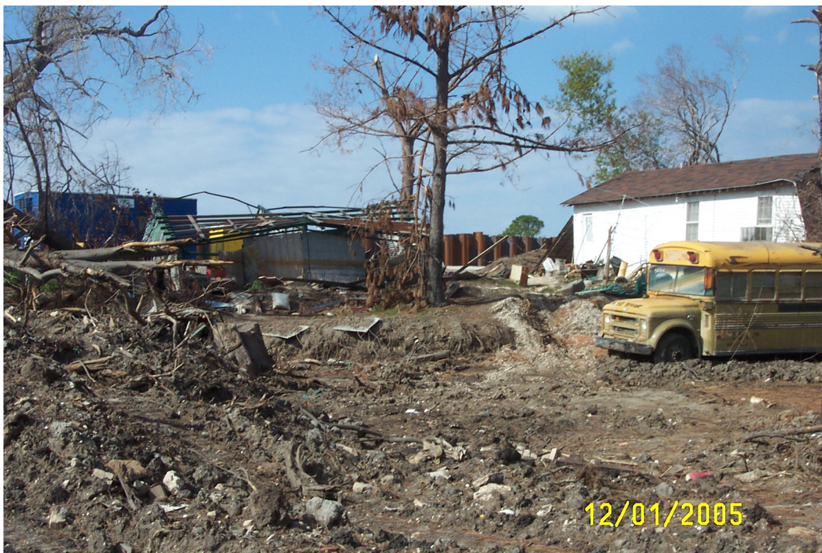
Figure 38. . Slide toe (at abrupt change in slope in front of school bus) where levee and neighborhood were displaced about 45 feet toward the viewer.
