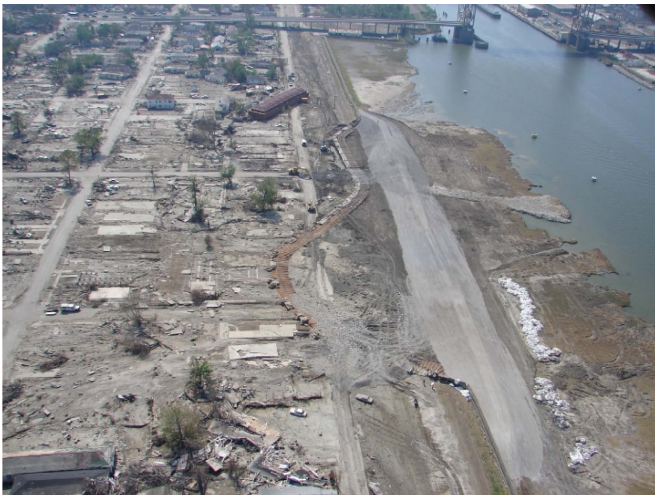
Figure 14. View of southern breach on the Industrial Canal, looking South. Note the floodwall and sheet piling (brown) strewn through the Lower Ninth Ward neighborhood where all houses were removed by the force of water coming through the breach. Gray deposits on right are breach repair gravels. Note barge near in the center near the top of the photo. Photo by L. Harder - Independent Levee Investigation Team Draft Final Report (2006).
