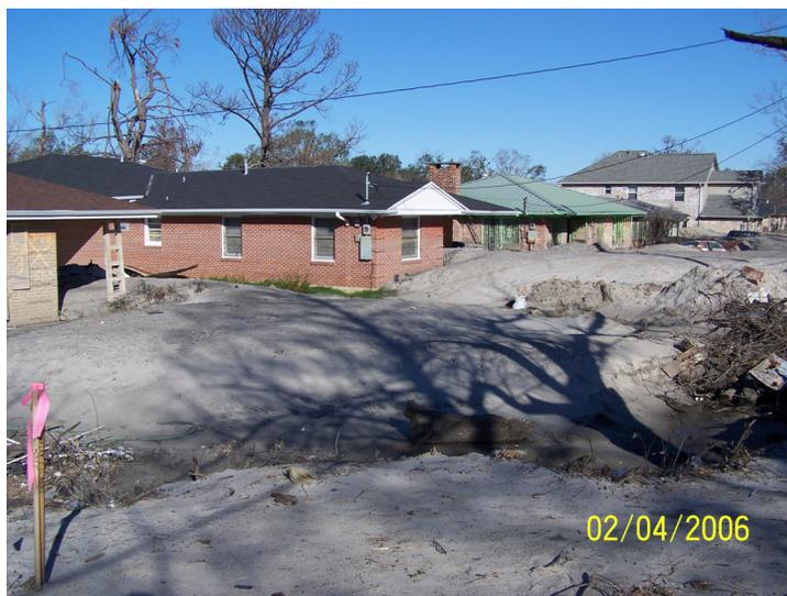
**Figure 19.** Sand deposits on Warrington drive showing deposition in the wake of houses as the currents flowed down the driveways between the houses. As of March 1, 2006, most of the sand deposits have been removed.
