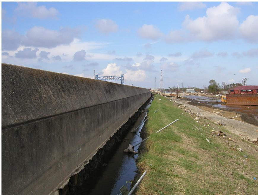
**Figure 11.** Looking North along the floodwall of the Industrial Canal levee showing trenches eroded by water from the Industrial Canal that overtopped the floodwall. Photo from U.S. Army Corps of Engineers IPET web site, taken October 4, 2005.
