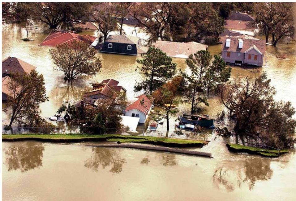
Figure 42. View of 17 th St. Canal breach looking toward east. Note fractures in the displaced part of the levee. Photo by J. Augustino FEMA.
