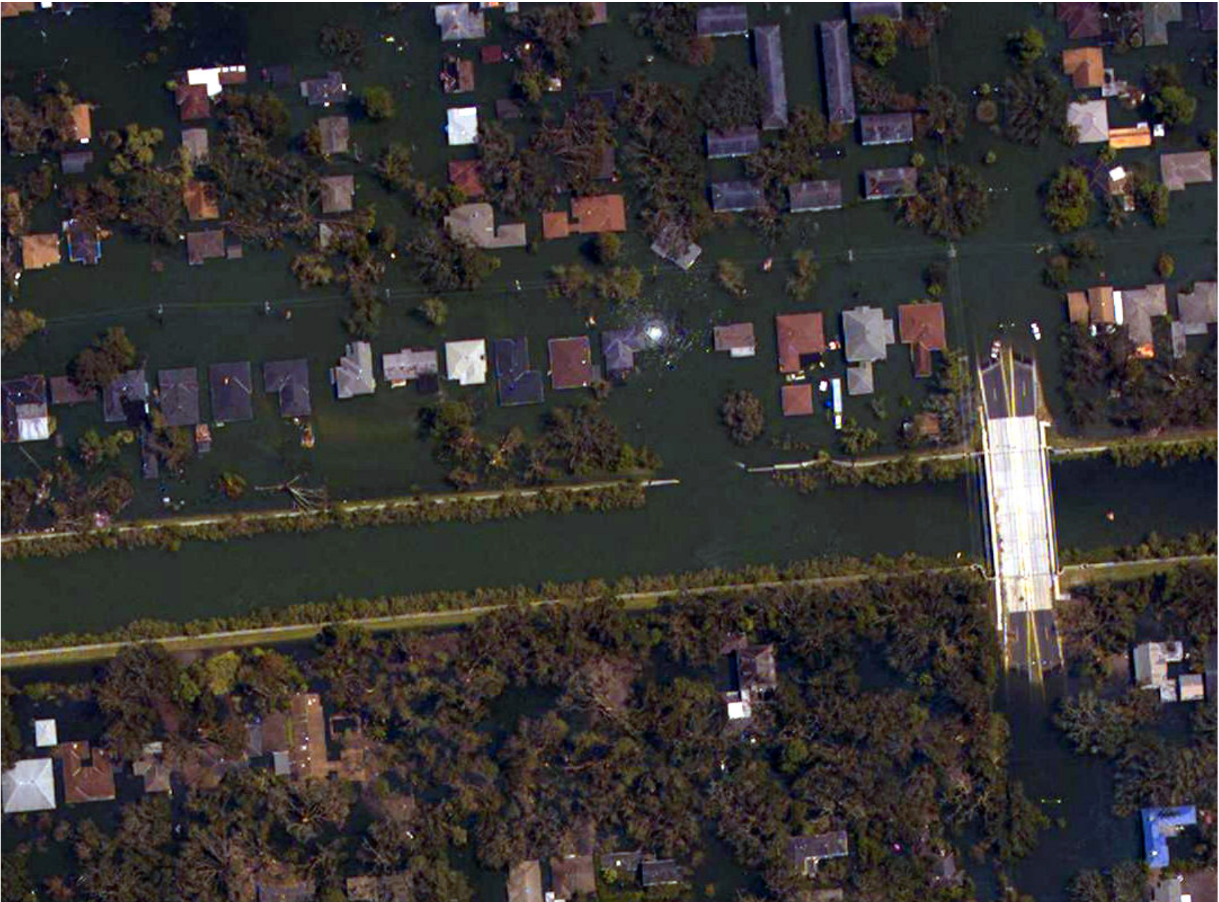
Figure 26. Air photograph of the area where the London Avenue Canal levee was breached near Mirabeau Ave. and Warrington Drive (Stop 4). Image acquired Aug. 31, 2005. Source: National Oceanic and Atmospheric Administration's National Geodetic Survey, Katrina Images - http://ngs.woc.noaa.gov/katrina/
