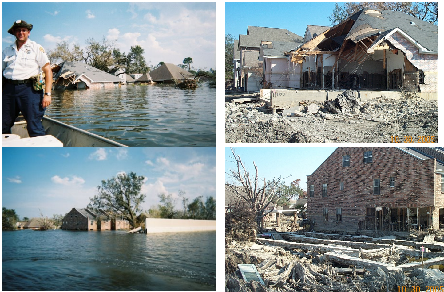
Figure 49. Comparison of water levels on Sept.1, 2005 (photos on left by Kevin Himmel), with water lines on same structures indicate lines left by standing water are about 1.5 to 2 feet lower than the maximum water level. Note large block of peat in photo at the upper right. In photo at lower right, note the chainwall foundation of a house that was removed by the burst of water when the levee was breached and the cypress stump from a tree that was probably cut down 100 years ago when this Lakeview neighborhood was reclaimed from the cypress swamp.
