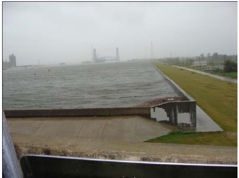
Figure 23. View of the Industrial Canal from the Claiborne Ave. Bridge looking North toward Stop 7 with the Florida Ave. Bridge (blue bridge) on the horizon. Photo as taken on the morning of Sept. 1, 2008 during the passage of Hurricane Gustav. Note the elevation drop from the post-Katrina floodwall (on the right) to the original floodwall to the left. Photo from U.S. Army Corps of Engineers.
