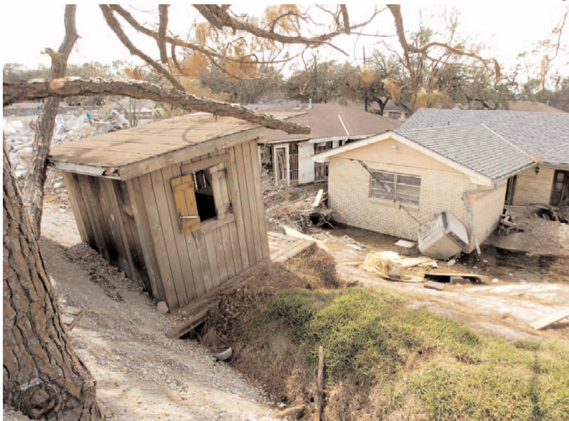
Figure 35. Child's clubhouse behind the Cantrell home on Pratt Drive uplifted along the west side of the London Avenue Canal near the breach (Stop 5). Note the fractures beneath and in front of (right side in photo) the clubhouse. Gray material at base of tree is gravel used in the repair of the breach. Source: Times-Picayune Tuesday, October 4, 2005. See reference to article by John McQuaid, same date
