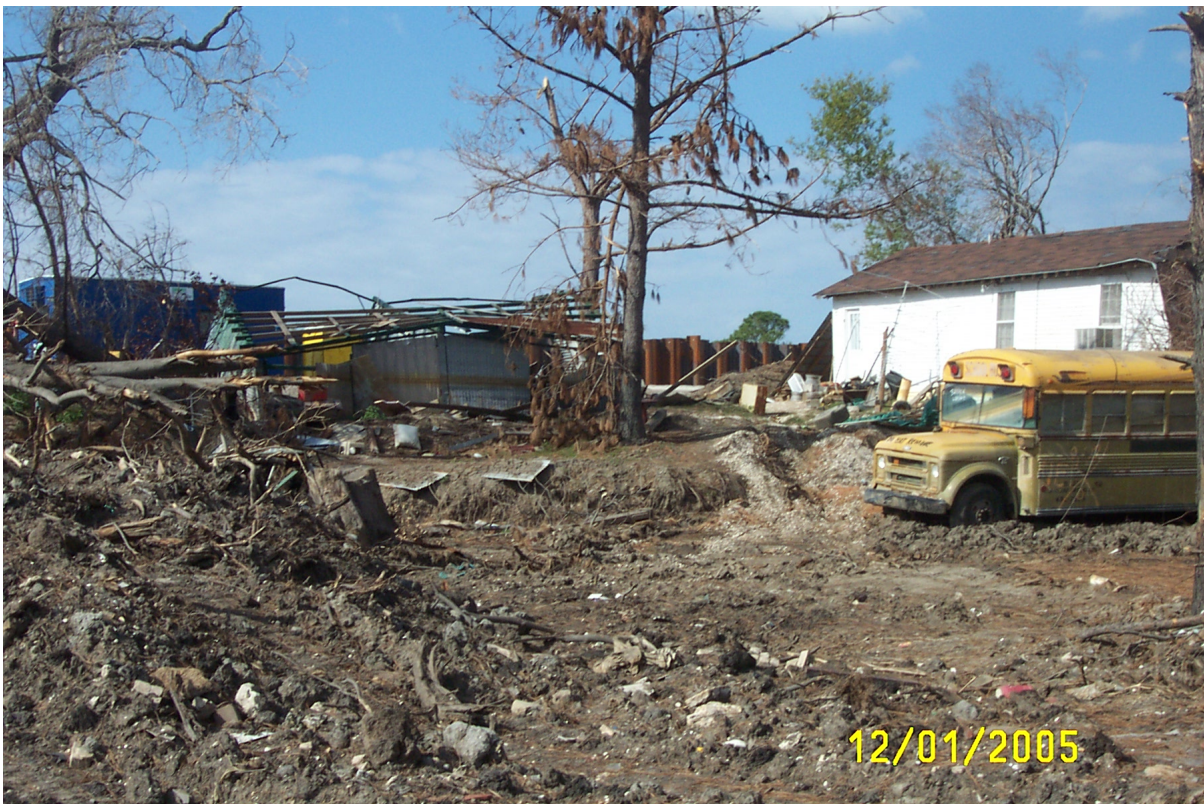
Figure 43. Slide toe (at abrupt change in slope in front of school bus) where levee and neighborhood were displaced about 45 feet toward the viewer.
