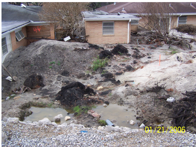
Figure 37. Sand deposits and peat blocks (black) behind homes on Pratt Drive at the North breach of the London Ave. Canal. Note the sand boil on the right. Gray material in the foreground is gravel used in the repair of the breach.
