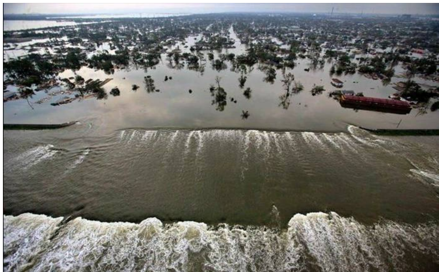
Figure 13. The large breach in the Industrial canal that flooded the Lower Ninth Ward could have been caused by a barge crashing through the floodwall during Katrina. Alternatively the barge could have floated in after the levee and floodwall were breached. Note the barge in the photo above. Note also that at the time of this photo water was running out of the Lower Ninth Ward back into the Industrial Canal. (Source - Vincent Laforet, AFP/Getty Images)
