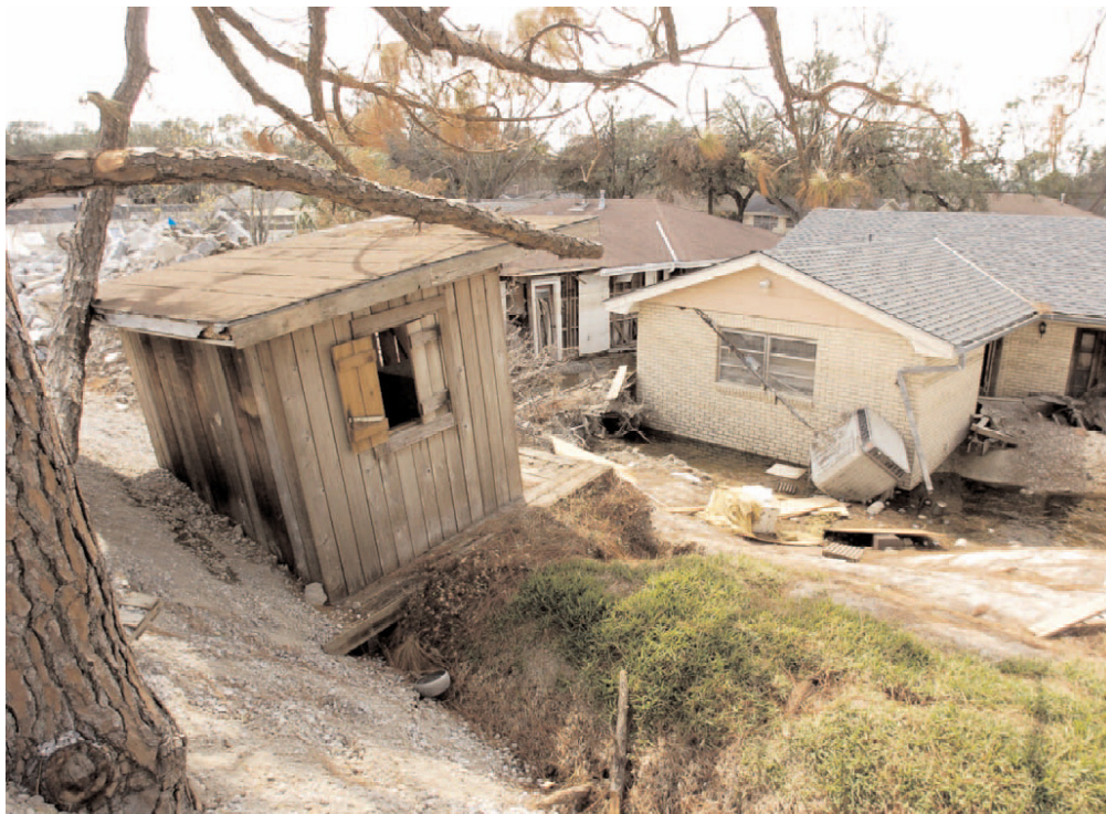
Figure 27. Child's clubhouse behind the Cantrell home on Pratt Drive uplifted along the west side of the London Avenue Canal near the breach (Stop 3). Source: Times-Picayune Tuesday, October 4, 2005. See reference to article by John McQuaid, same date
