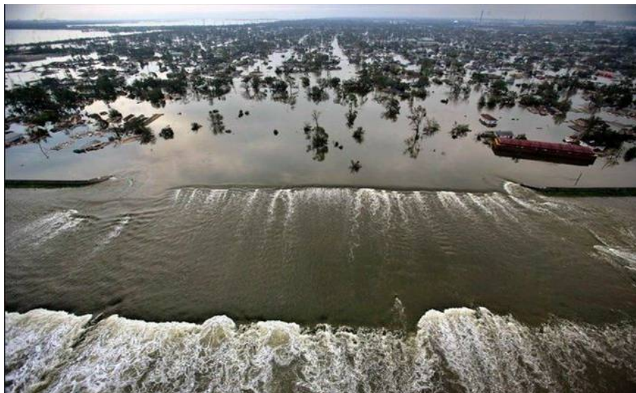
Figure 8. The large breach in the Industrial canal that flooded the Lower Ninth Ward could have been caused by a barge crashing through the floodwall during Katrina. Alternatively the barge could have floated in after the levee and floodwall were breached. Note the barge in the photo above. Note also that at the time of this photo water was running out of the Lower Ninth Ward back into the Industrial Canal. (Source - Vincent Laforet, AFP/Getty Images)
