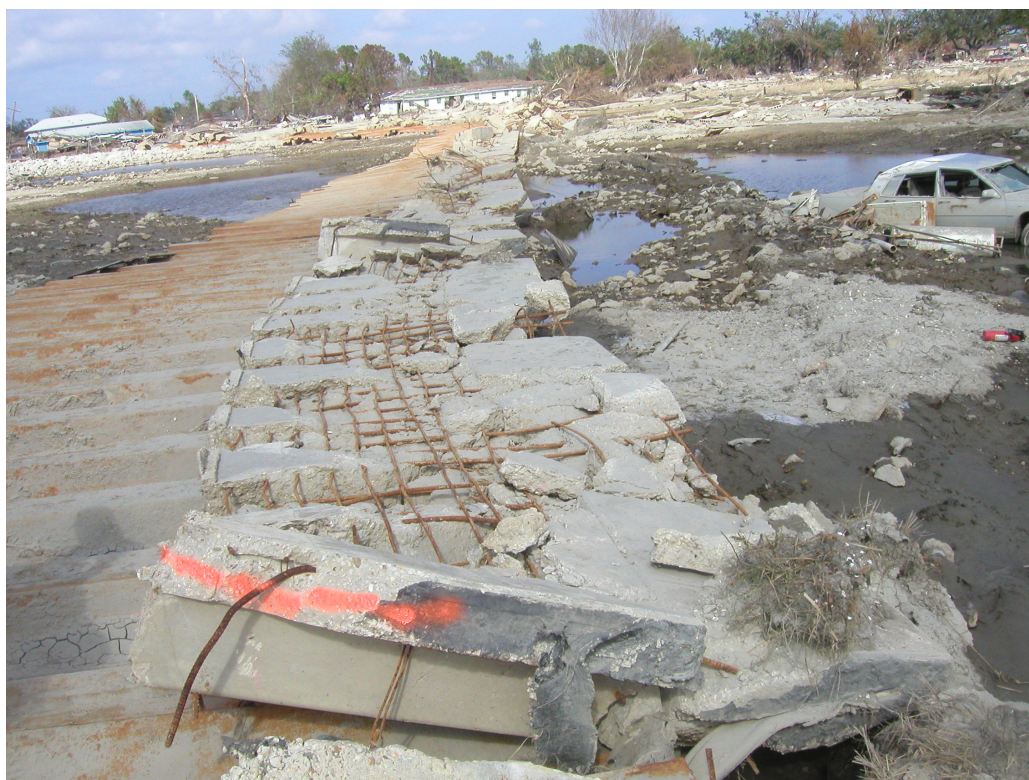
Figure 12. Floodwall and sheet piling strewn into Lower 9 th Ward at the southern (larger) breach on the Industrial Canal. Photo from U.S. Army Corps of Engineers IPET web site, taken October 4, 2005.
