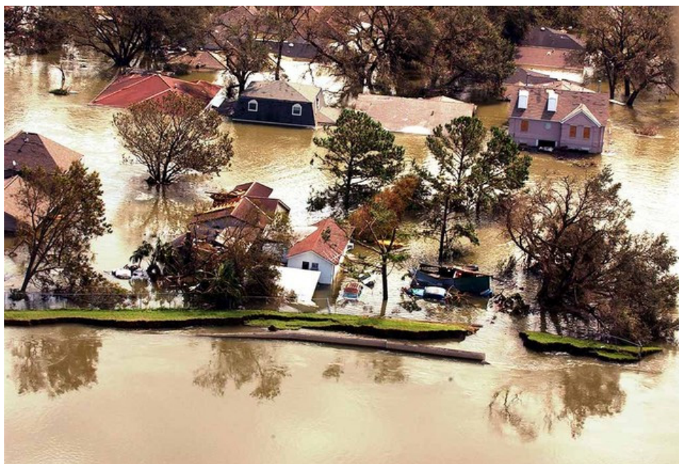
Figure 32. View of 17 th St. Canal breach looking toward east. Note fractures in the displaced part of the levee. Photo by J. Augustino FEMA.
