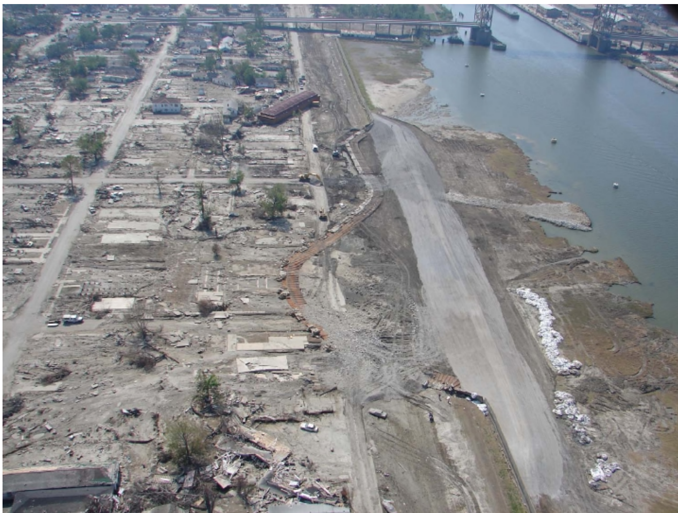
Figure 13. View of southern breach on the Industrial Canal, looking South. Note the floodwall and sheet piling (brown) strewn through the Lower Ninth Ward neighborhood where all houses were removed by the force of water coming through the breach. Gray deposits on right are breach repair gravels. Note barge near in the center near the top of the photo. Photo by L. Harder - Independent Levee Investigation Team Draft Final Report (2006).
