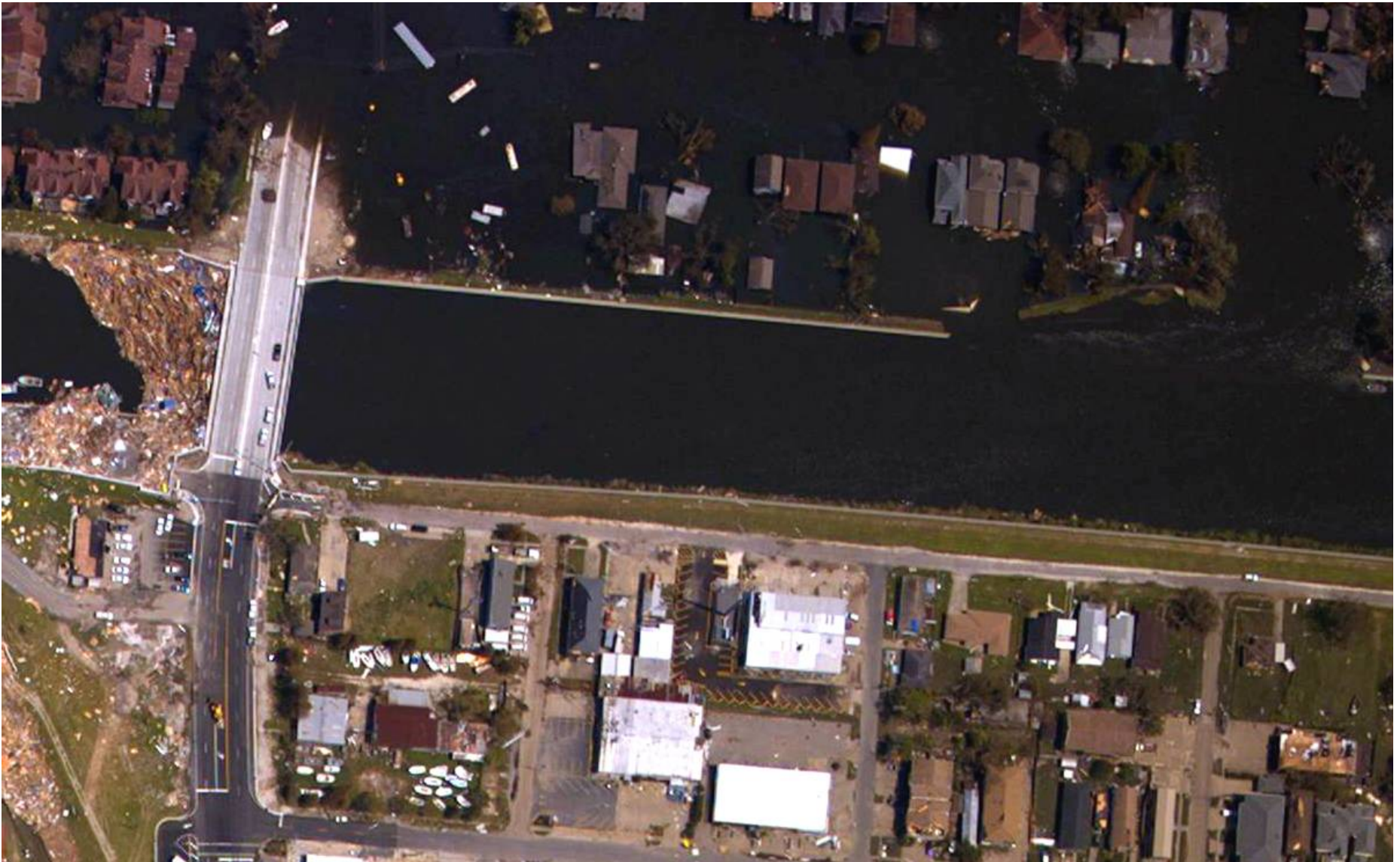
Figure 30. Air photograph of the area where the 17th Street Canal Levee was breached near Belaire Drive (stop 5). Image acquired Aug. 31, 2005. Source: National Oceanic and Atmospheric Administration's National Geodetic Survey, Katrina Images - http://ngs.woc.noaa.gov/katrina/
