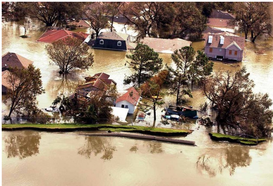
Figure 32. View of 17 th St. Canal breach looking toward east. Note fractures in the displaced part of the levee.
