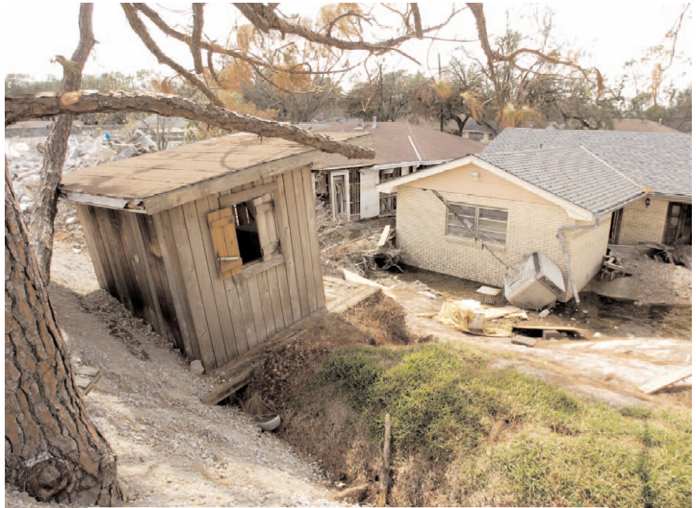
Figure 27. Child's clubhouse behind the Cantrell home on Pratt Drive uplifted along the west side of the London Avenue Canal near the breach (Stop 2). Source: Times-Picayune Tuesday, October 4, 2005. See reference to article by John McQuaid, same date
