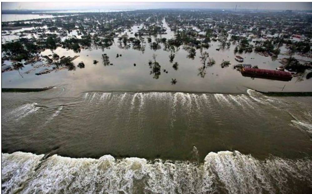
Figure 8. The large breach in the Industrial canal that flooded the Lower Ninth Ward could have been caused by a barge crashing through the floodwall during Katrina. Alternatively the barge could have floated in after the levee and floodwall were breached. Note the barge in the photo above. Note also that at the time of this photo water was running out of the Lower Ninth Ward back into the Industrial Canal. (Source - Vincent Laforet, AFP/Getty Images)
