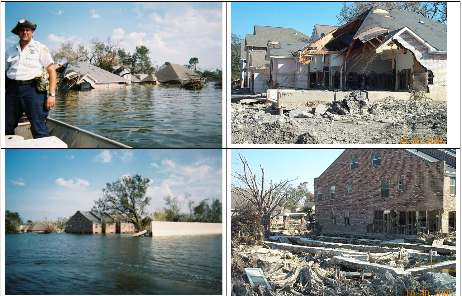
Figure 38. Comparison of water levels on Sept. 1, 2005 (photos on left by Kevin Himmel), with water lines on same structures indicate lines left by standing water are about 1.5 to 2 feet lower than the maximum water level. Note large block of peat in photo at the upper right. In photo at lower right, note the chainwall foundation of a house that was removed by the burst of water when the levee was breached and the cypress stump from a tree that was probably cut down 100 years ago when this Lakeview neighborhood was reclaimed from the cypress swamp.
