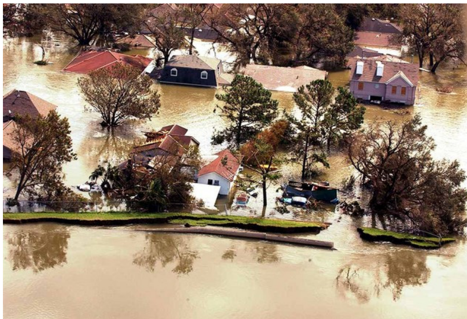
Figure 41. View of 17 th St. Canal breach looking toward east. Note fractures in the displaced part of the levee. Photo by J. Augustino FEMA.
