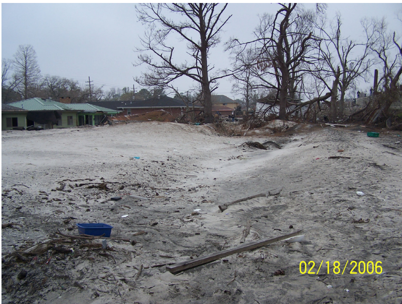
Figure 26. Sand deposits near the south breach of the London Avenue canal. (a) sand ridges deposited in the wake of houses as the currents flowed down the driveways between the houses. (b) Sand deposits that buried two cars in front of house on Warrington Drive . (c) Ridges of sand filling the back yards of houses along Warrington Drive, just north of the breach. As of March 1, 2006, most of the sand in the front yards had been removed and as of mid January, 2007 most of the sand in the backyards had been removed.
