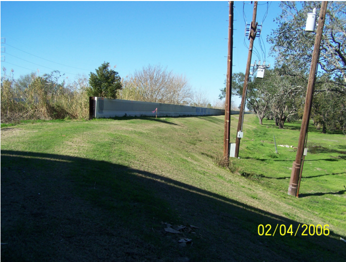
Figure 50. End of floodwall on Orleans Canal just north of I-610 overpass near Marconi Ave. (Stop 6)
