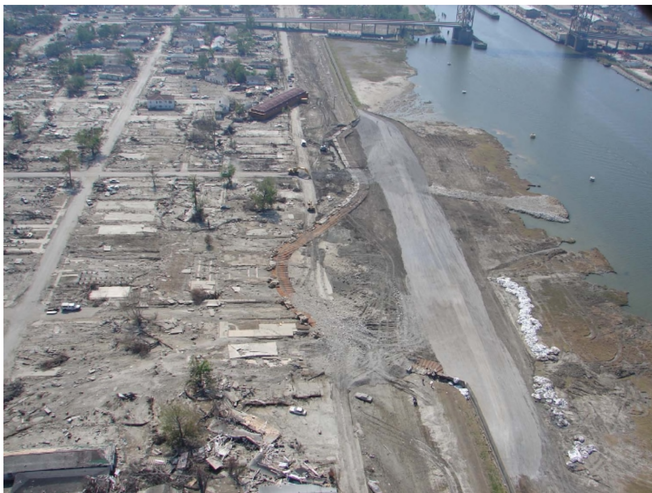
Figure 14. View of southern breach on the Industrial Canal, looking South. Note the floodwall and sheet piling (brown) strewn through the Lower Ninth Ward neighborhood where all houses were removed by the force of water coming through the breach. Gray deposits on right are breach repair gravels. Note barge near in the center near the top of the photo. Photo by L. Harder - Independent Levee Investigation Team Final Report (2006).
