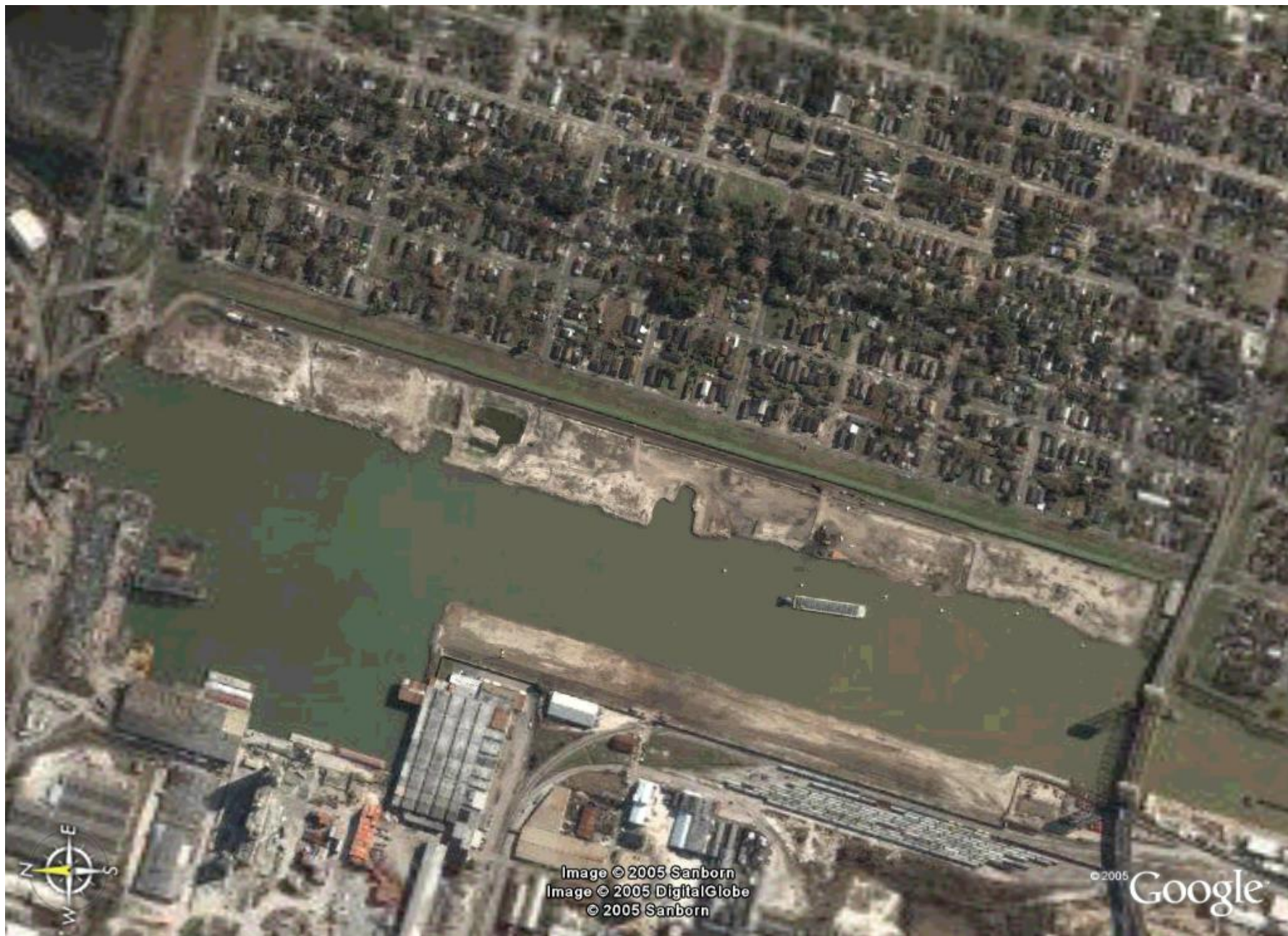
Figure 10. Satellite image of the area along the Industrial Canal where the levee was later breached during Hurricane Katrina. (Source - Google Earth)
