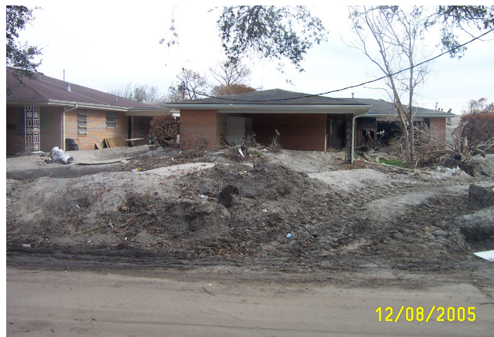
Figure 37. Sand deposits in front of houses on Pratt Drive at the North breach of the London Ave. Canal.
