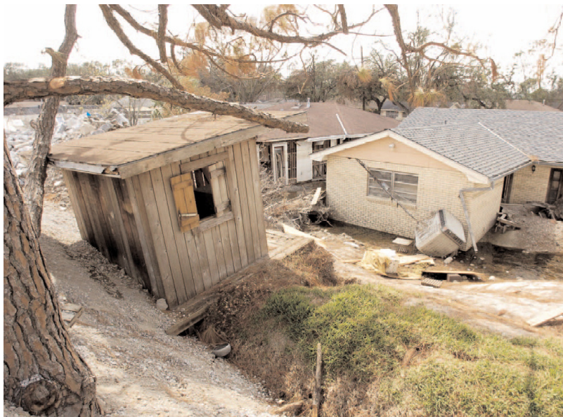
Figure 34. Child's clubhouse behind the Cantrell home on Pratt Drive uplifted along the west side of the London Avenue Canal near the breach (Stop 3). Note the fractures beneath and in front of (right side in photo) the clubhouse. Gray material at base of tree is gravel used in the repair of the breach. Source: Times-Picayune Tuesday, October 4, 2005. See reference to article by John McQuaid, same date
