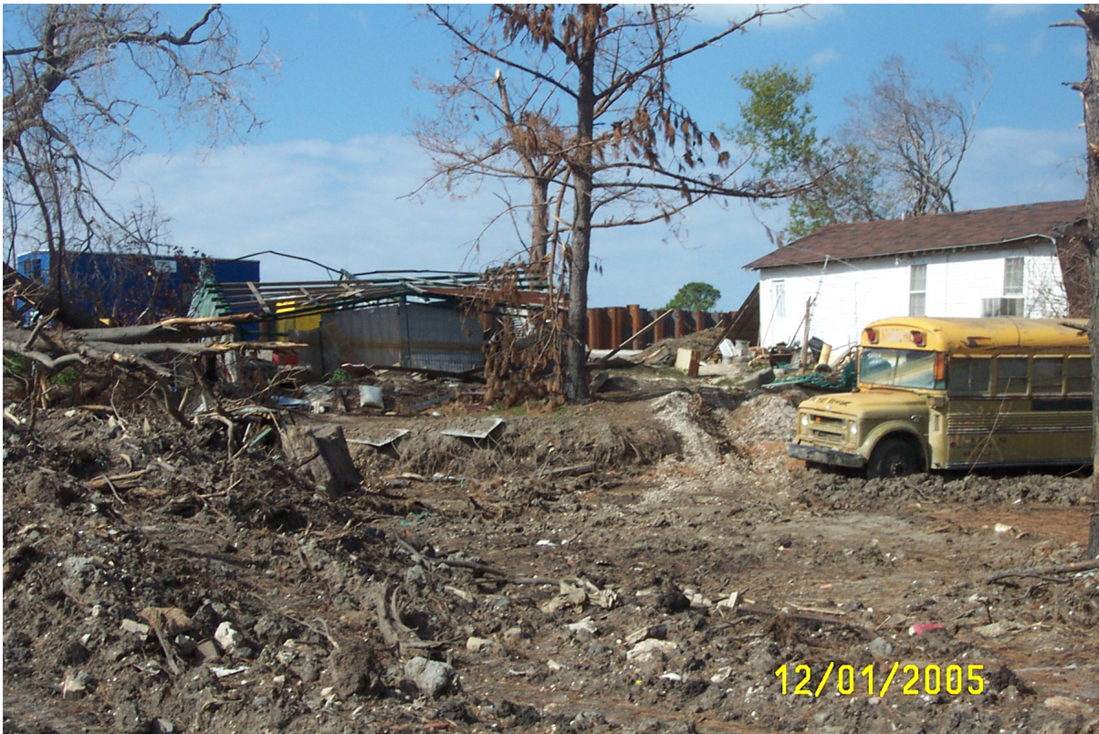
Figure 42. . Slide toe (at abrupt change in slope in front of school bus) where levee and neighborhood were displaced about 45 feet toward the viewer.
