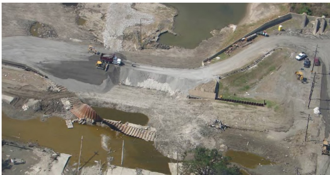
Figure 16. Aerial view of the north breach on Industrial Canal. Photo by L. Harder - Independent Levee Investigation Team Final Report (2006).
