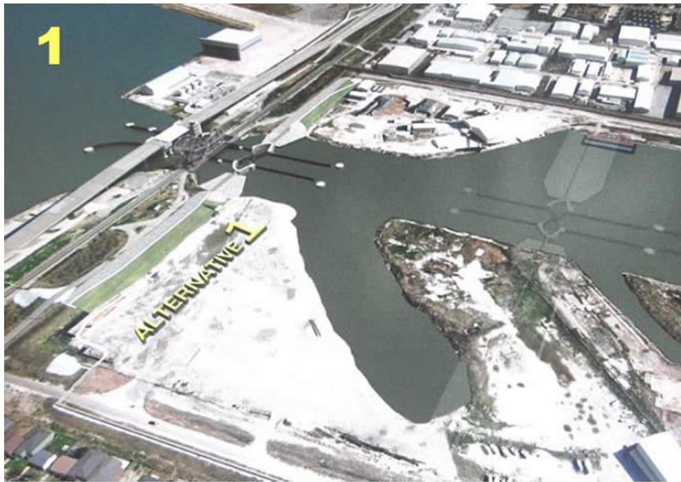
Figure 13 (From U.S. Army Corps of Engineers)
