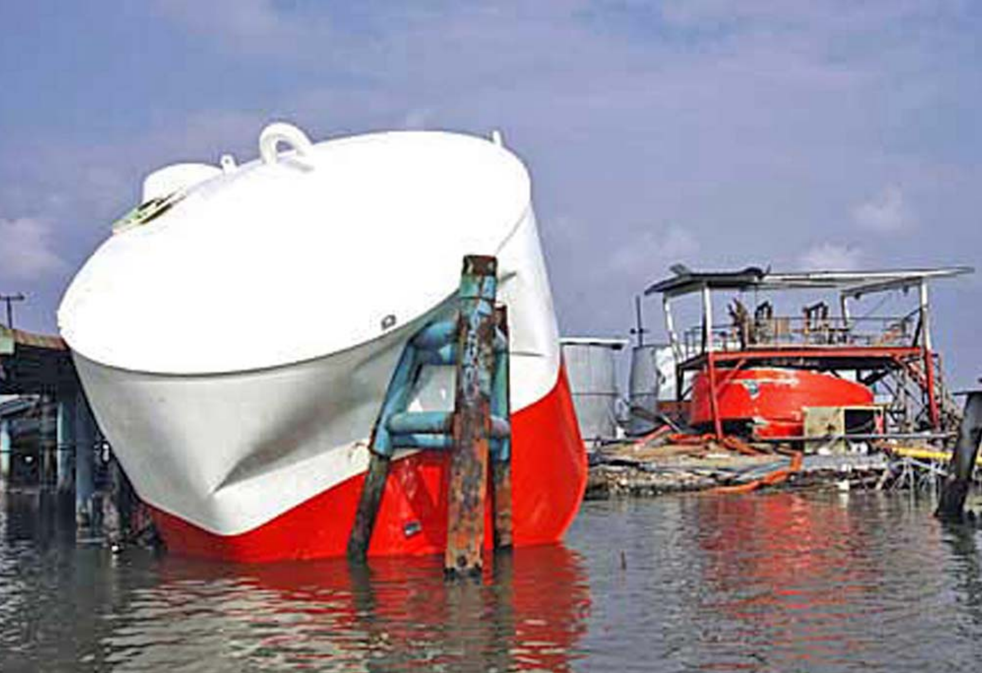
Oil facility in Cameron LA damaged
