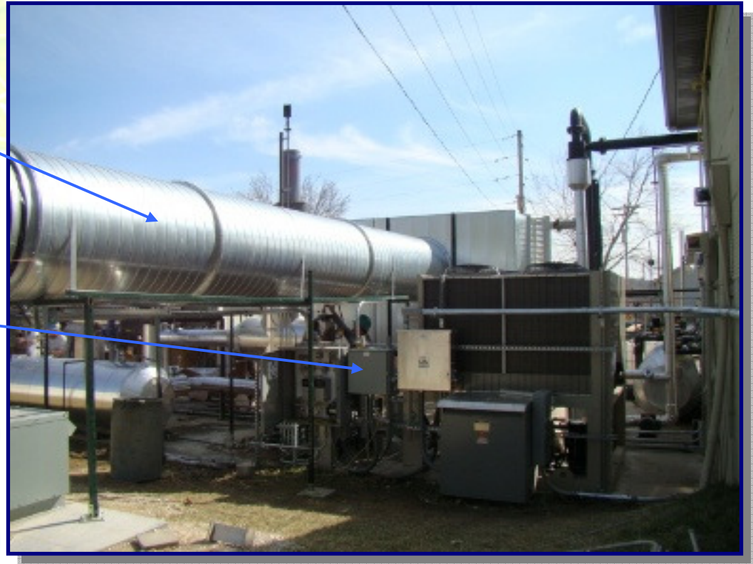
Rear view of syngas cooler
