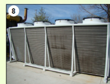
Cogeneration heat exchanger
