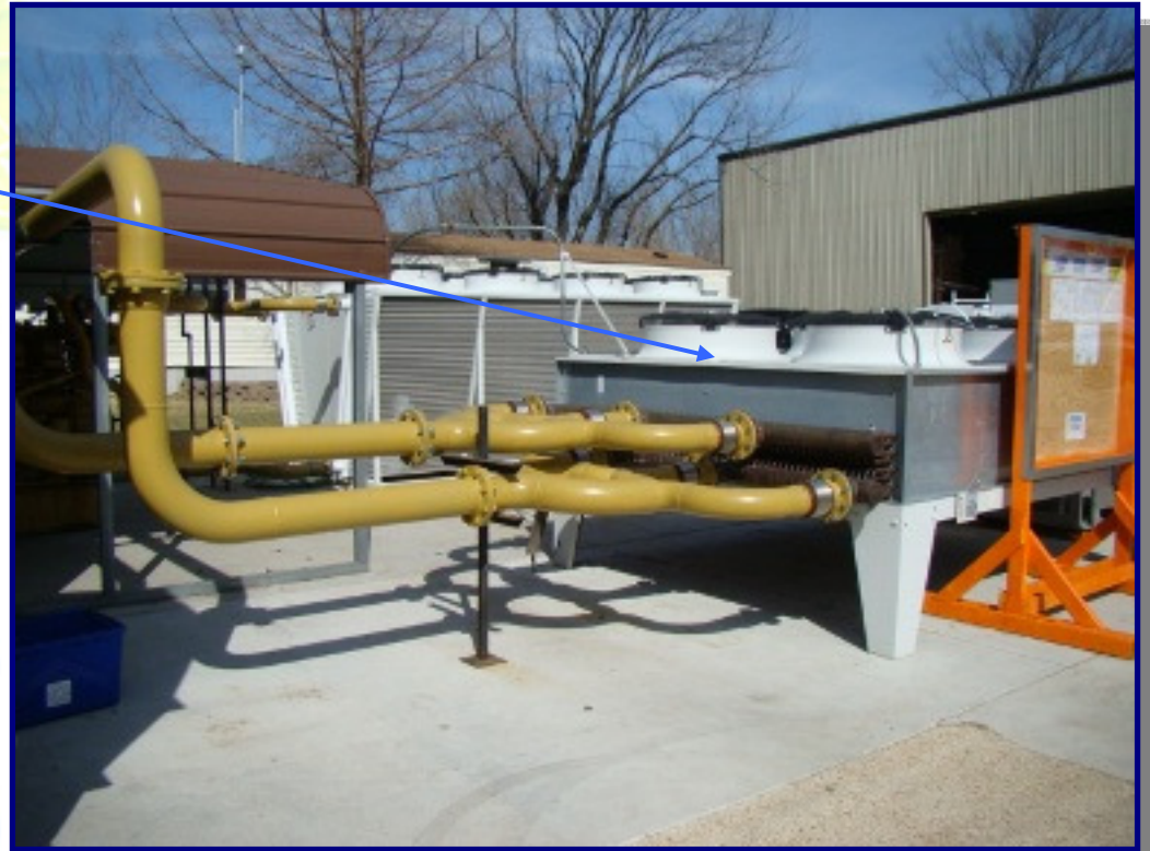
Turbocharger after cooler
