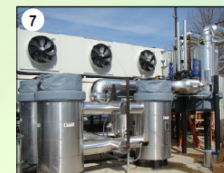
Syngas cooler and filter
